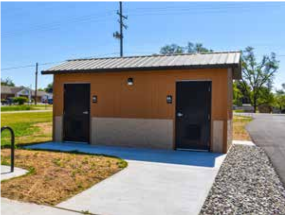
Mill Pond Park features a two-stall unisex prefabricated restroom with full utilities.
