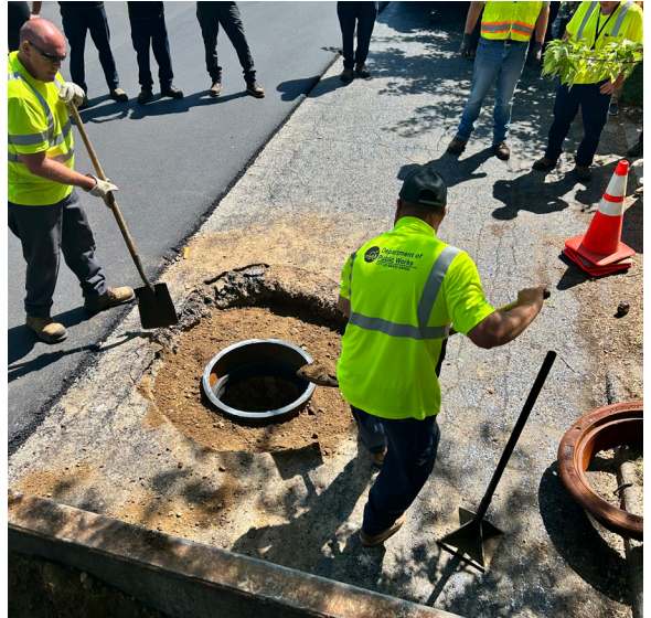
DPW employees participate in manhole demo
