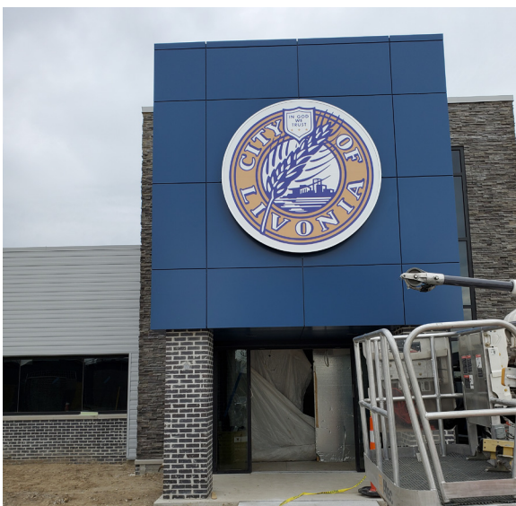
The new City of Livonia DPW building
