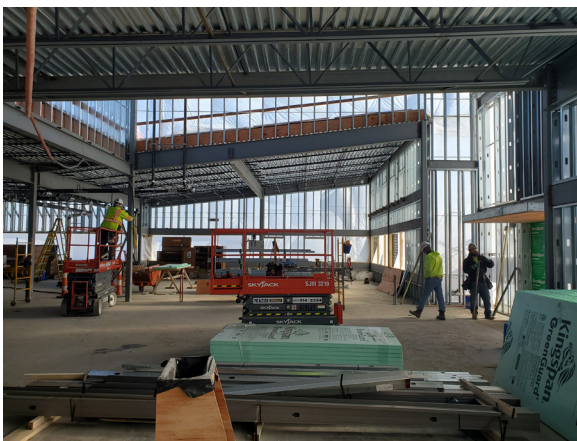
Construction of the new DPW building
