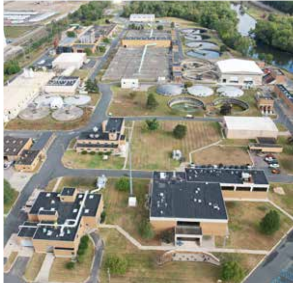
Aerial view of the Kalamazoo Water Reclamation Plant
