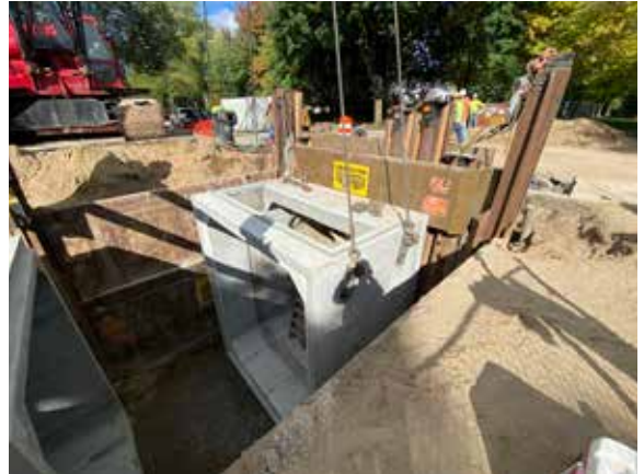
Downstream end of outlet control structure
