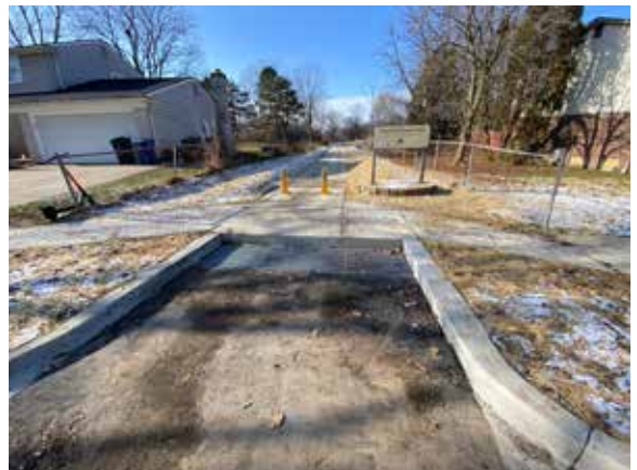
Downstream end of project, outlet control structure
