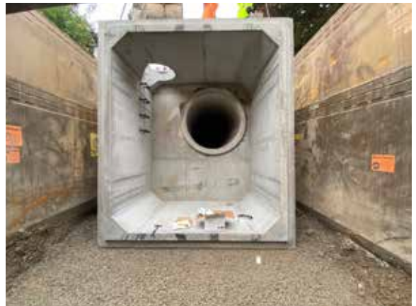
Inside of outlet control structure
