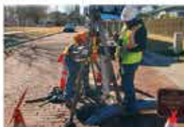
CURED-IN-PLACE PIPE
