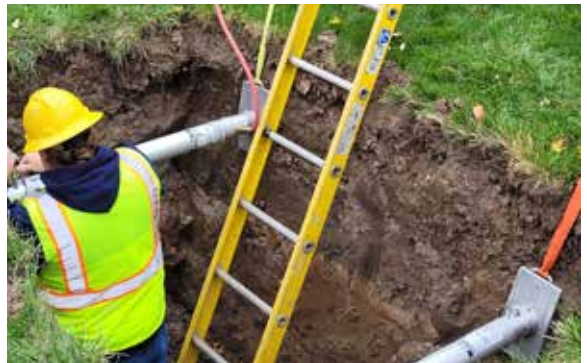
Trenching and Shoring Class
