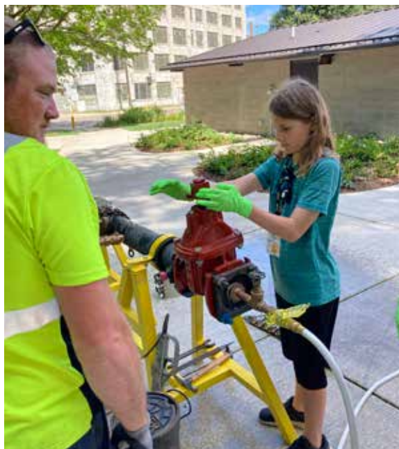
Camper opening a valve to check whether the water main repair was successful.
